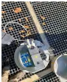
ISCO at Effluent
