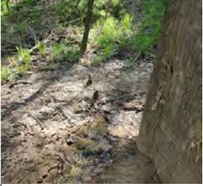
Upstream, some seeps in background not captured due to no channelized flow
