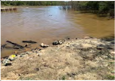
North side of ramp
