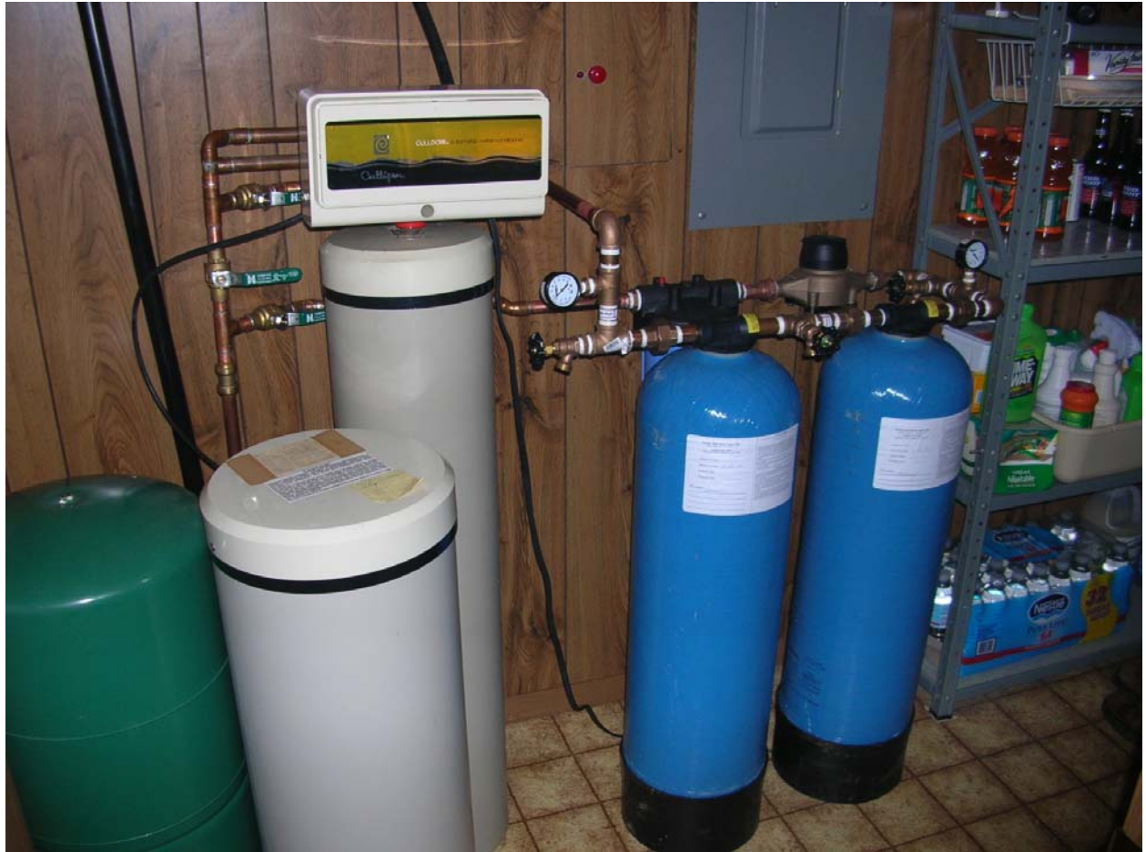
Photograph of a GAC System
