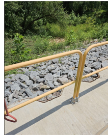
No water flow at outlet
