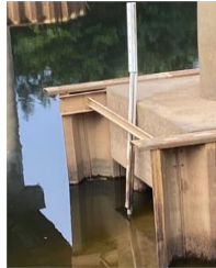
Staff gauge out of water
